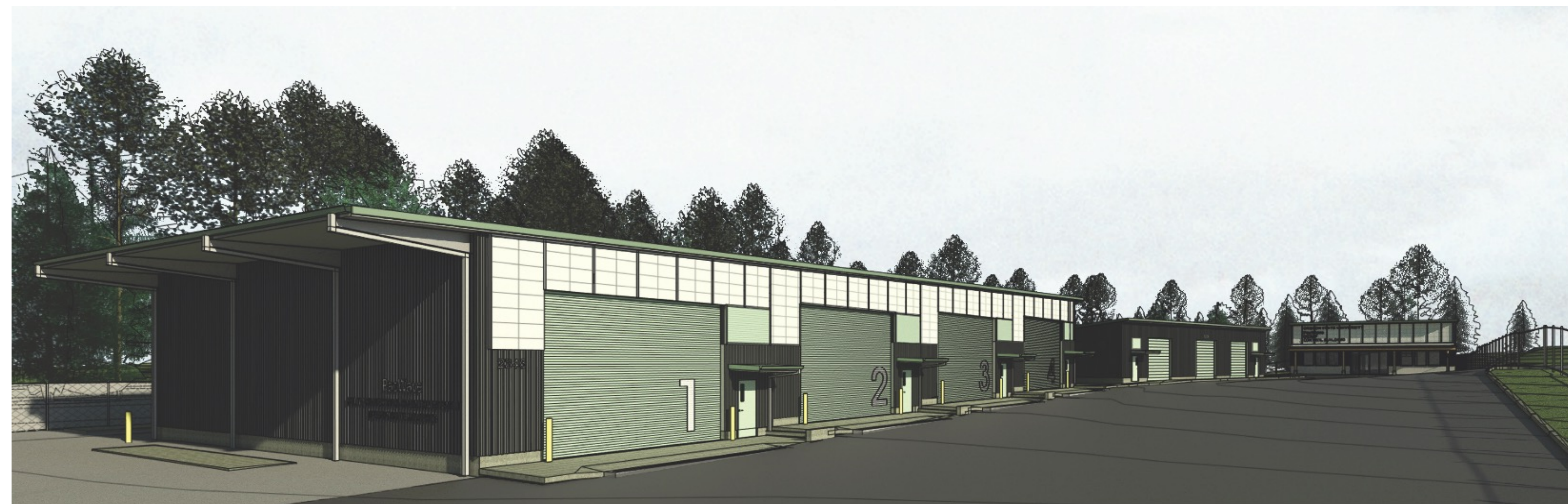
Shoreside Utility Connection and Monitoring Facility for grid integration research
