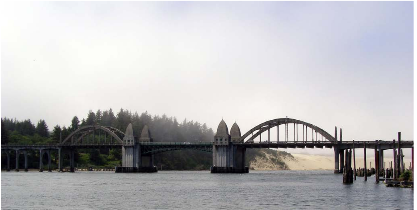
Figure 3 Image of a historical Siuslaw River Bridge at Florence.
