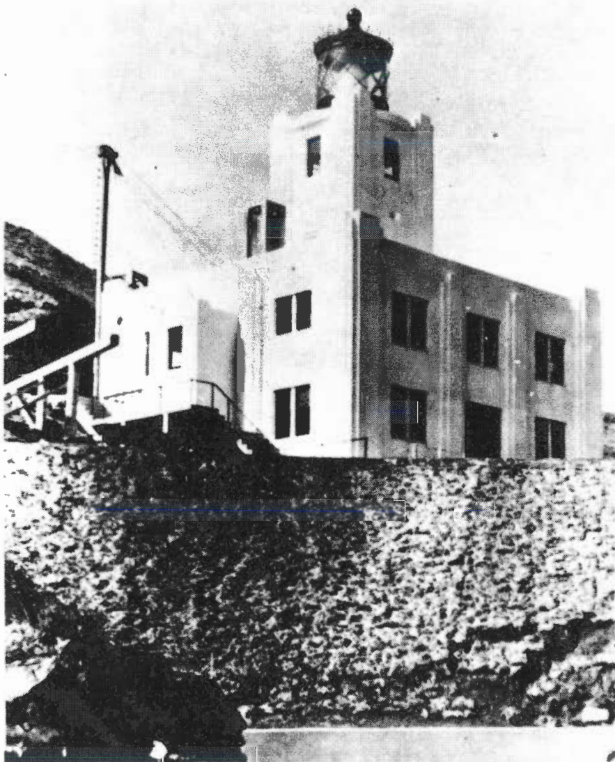
Scotch Cap Light Station, destroyed by Tsunami of 1946, killing all five occupants. Built in 1940 of concrete to replace a wooden structure built in 1903, it stood 60 feet high and 92 feet above water level. (Credit: U.S. Coast Guard.)
