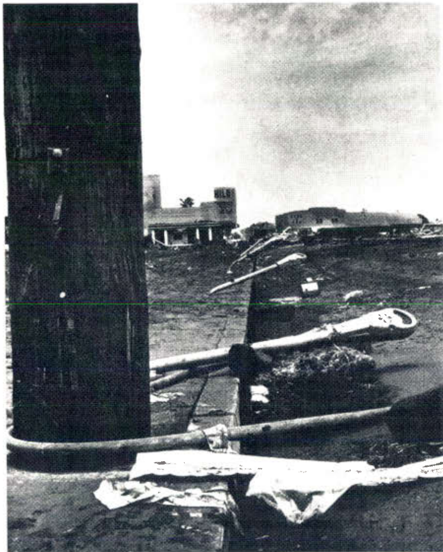
Tsunami of May 22, 1960, Hilo, Hawaii. flattened parking meters show direction and force of Tsunami.
